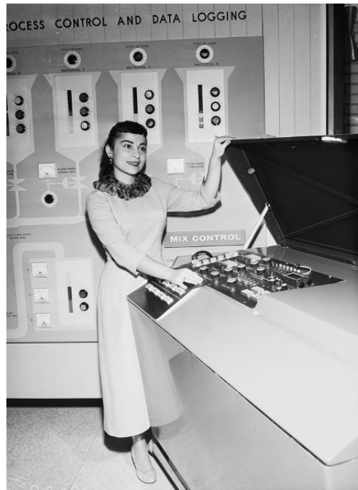
Figure 1.2 The picture of Ramo-Wooldridge (RW-300) computer used in process control and data logging
